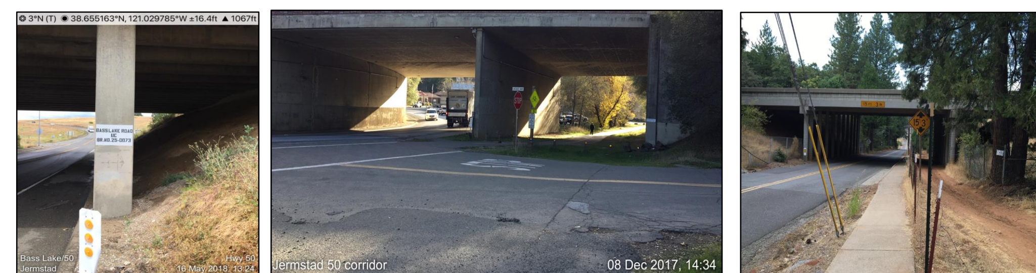
Existing overpasses on Highway 50 that are currently being used by wildlife
