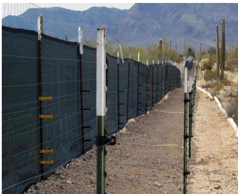
Figure 19: Hot-wire/ woven wire coyote enclosure with shade cloth for additional optical barrier Jill Bright AGFD
