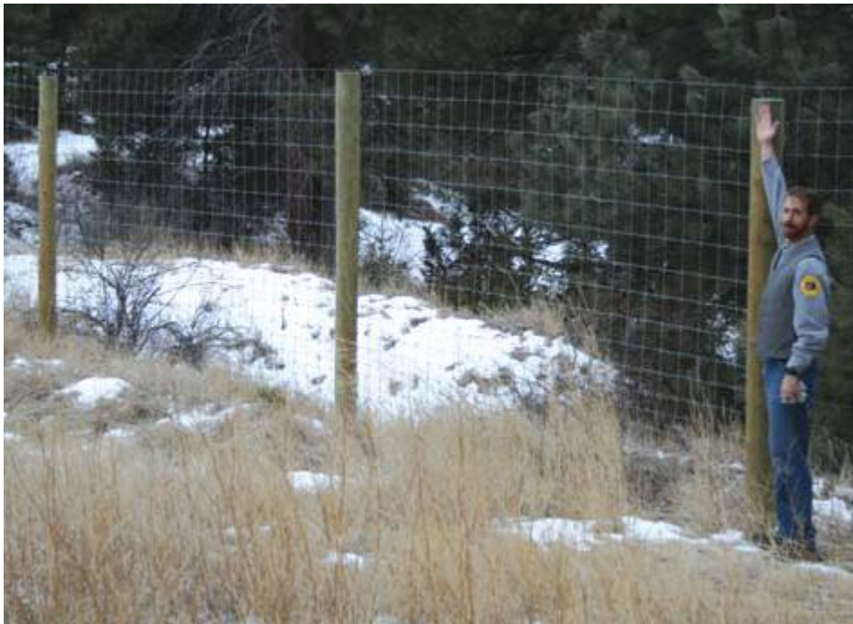
Figure 17: Eight foot woven wire fence
