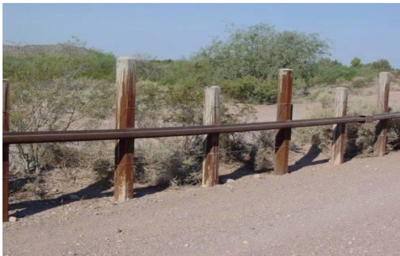
Figure 20: Post and rail vehicle barrier Duane Aubuchon, AGFD
